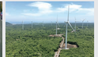
Onshore Wind Power (Jeju Gimnyeong Wind Power Complex)
