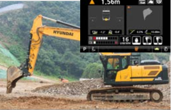
Effectiveness of earthworks improved by means of MC (Machine Control)
